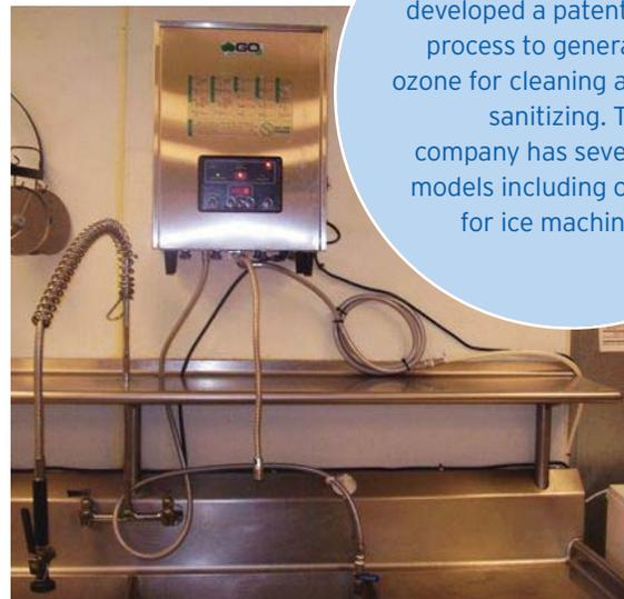
GO3 also has a unit specifically designed to provide water to ice machines (priced about \$4,000). Generating about 0.5 ppm of dissolved ozone, the water has just enough germ-killing efficacy to prevent bacterial growth in ice machines without altering the taste or odor of the ice itself. And unlike chlorine, which can badly corrode ice machine components, the ozonated water is perfectly safe.
